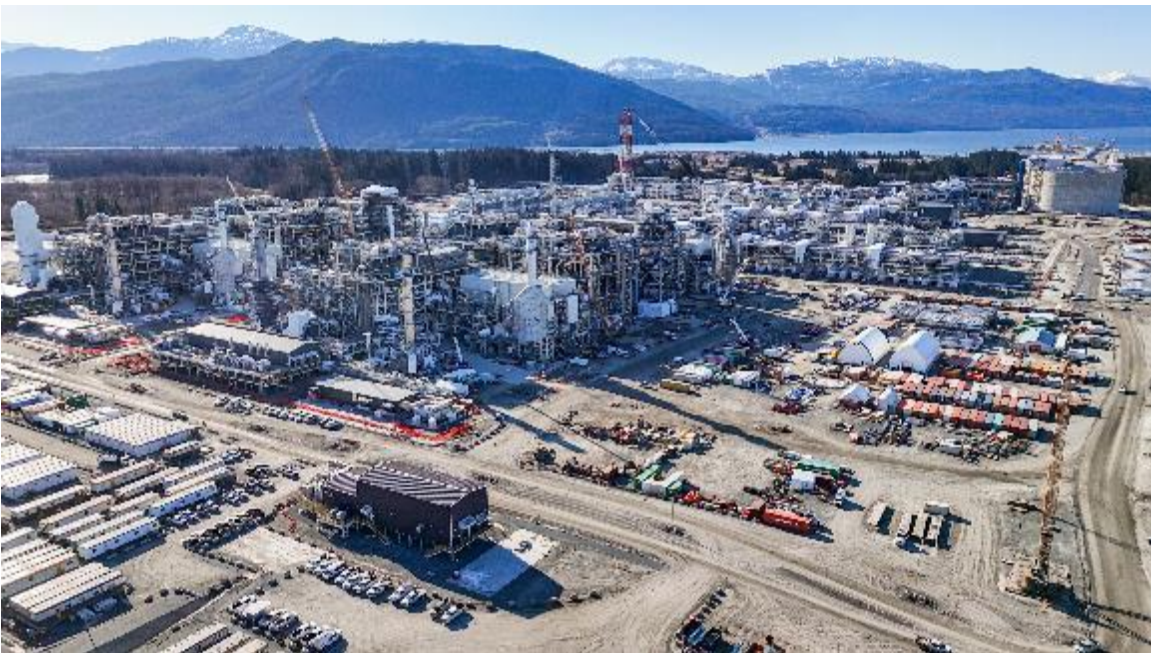
PHOTO 2: LNG FACILITY – VIEW OF THE LNG TRAINS TO THE NORTH (MARCH 2024)
