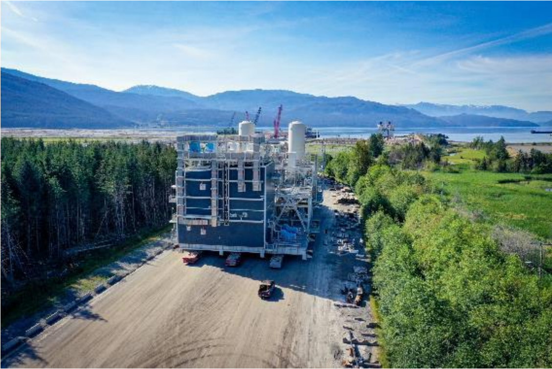
PHOTO 3: FINAL MODULE RECEIVED ON SITE (JULY 2023)
