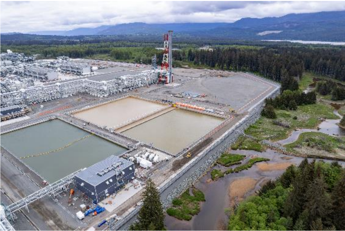
PHOTO 5: FLACK STACKS AND RETENTION BASINS
