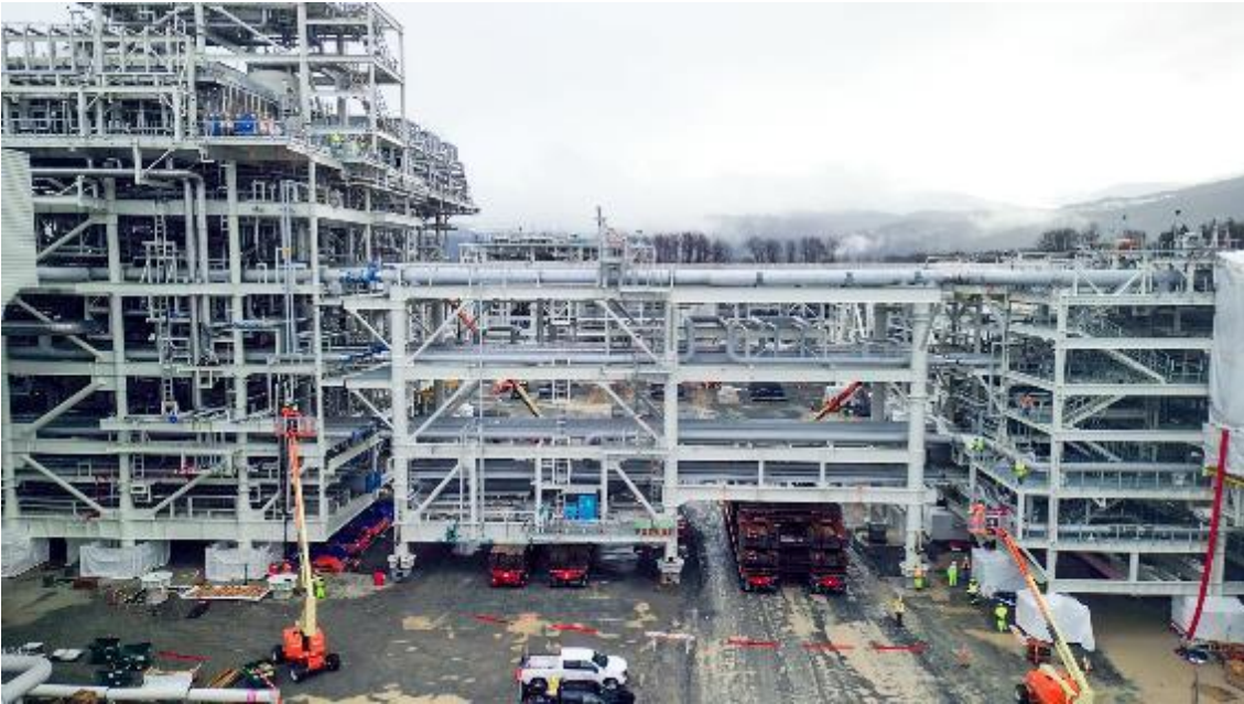
PHOTO 4: BRIDGE MODULE CONNECTING LNG TRAIN 1 TO UTILITIES (APRIL 2023)
