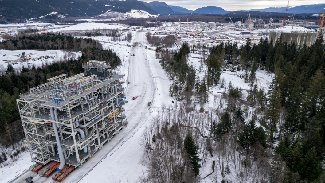
PHOTO 4: MODULE BEING MOVED TO THE FACILITY (JANUARY 2023)
