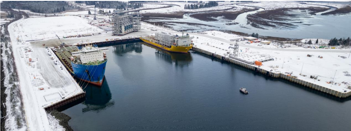
PHOTO 2: MODULE OFFLOAD AT THE MOF (DECEMBER 2022)
