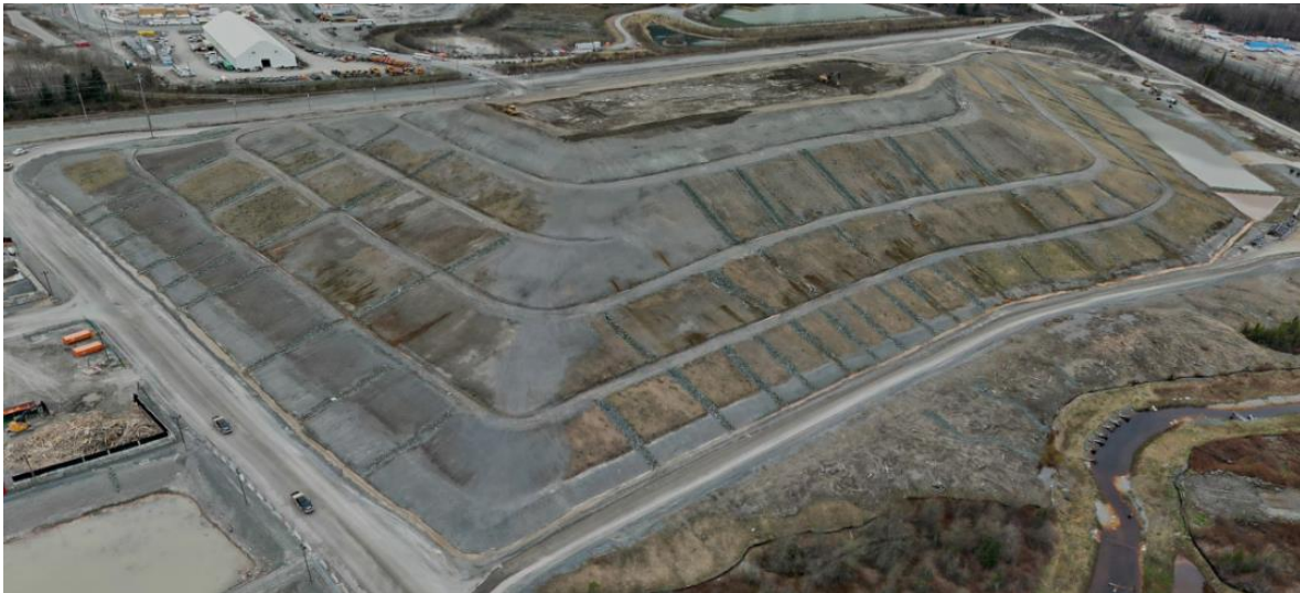
PHOTO 1: SOIL STOCKPILE (APRIL 2023)
